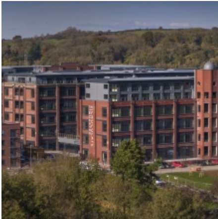
Advanced's MxPro 5 panels installed at The Chocolate Quarter
