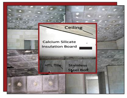
System 203<sup>m</sup> and System 203 Lite<sup>m</sup> is an interlocking refractor y tile and encapsulated insulating material. System 203<sup>m</sup> shields and protects training structures from the horrendous environments associated with live fire training. System 203<sup>m</sup> is able to withstand repeated high temperatures and extreme thermal shock created during fire extinguishment training evolutions without spalling, cracking, splintering or other degradation.
