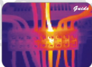
Inspect electricity hot point
