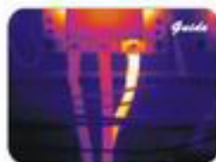
Inspect electricity hot point
