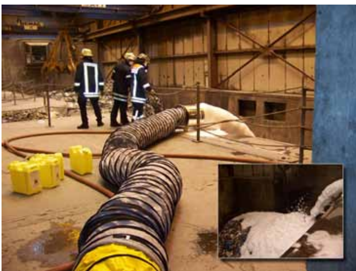
Foam covering in a waste incineration plant
